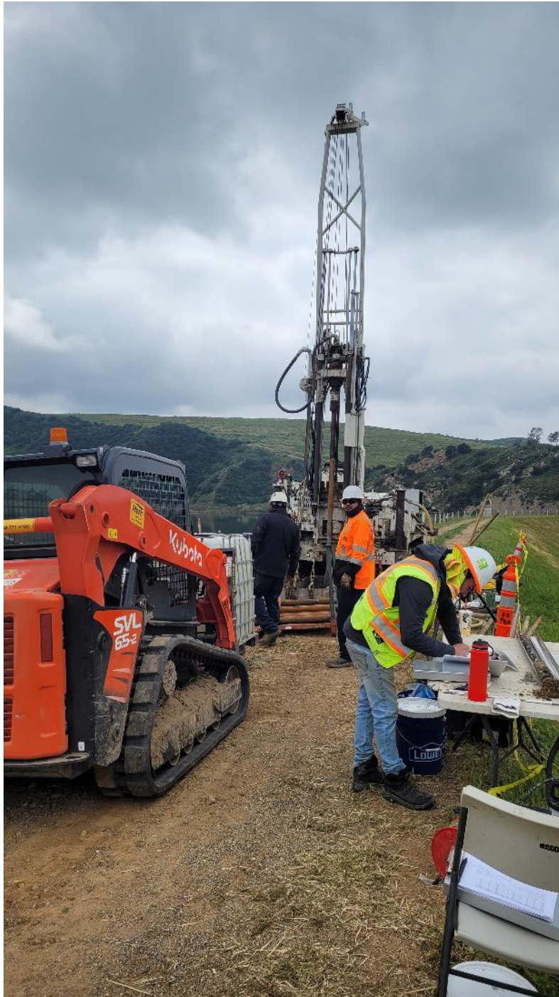
Photo 4: View of the ongoing geotechnical investigation.
