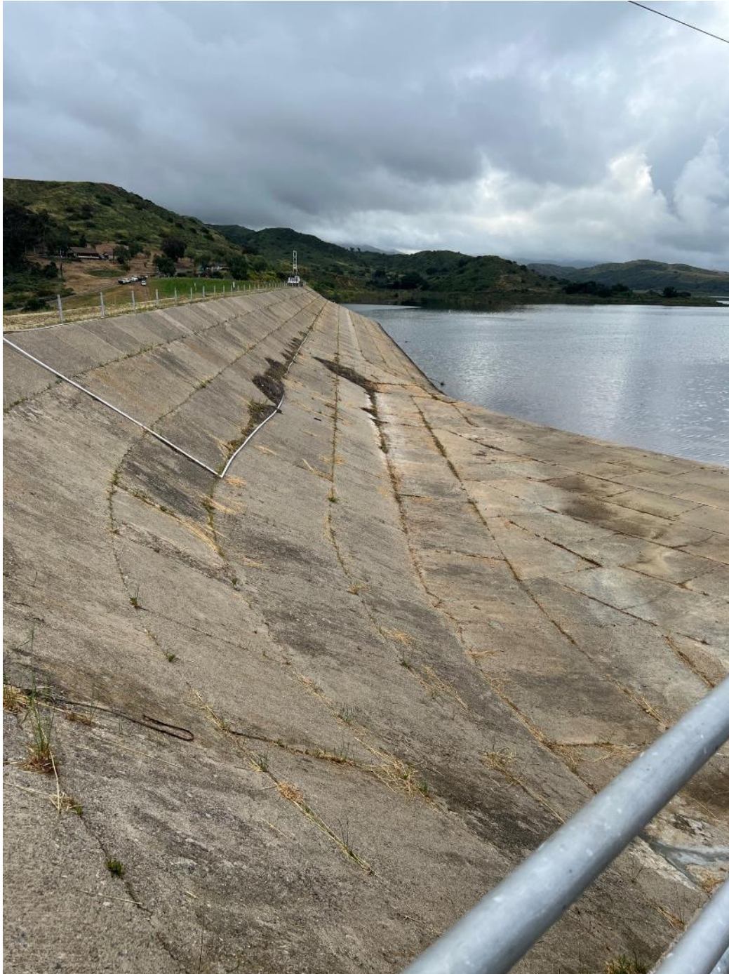
Photo 5: View of the cleared upstream slope. (Supplied by owner after inspection [5/3/2023]).
