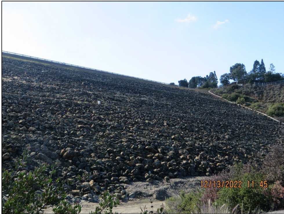
Photo 7) Downstream face looking towards left abutment.
