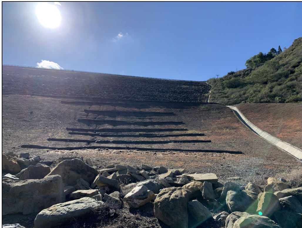
Photo 10) Looking upstream at left groin.
