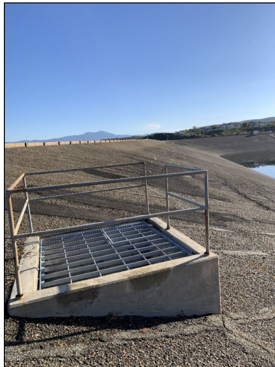
Photo 20) Close up of one (left) of the two spillways drop inlet structures located at upstream side of dam.
