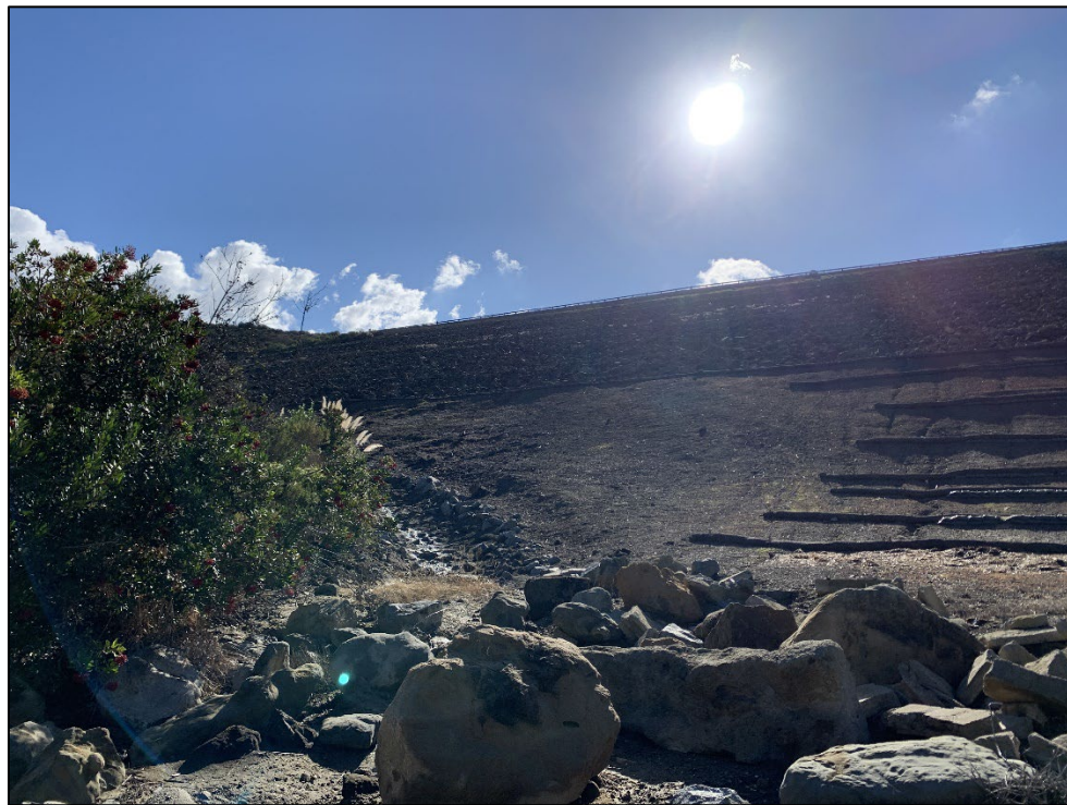
Photo 8) Downstream face looking at right abutment.
