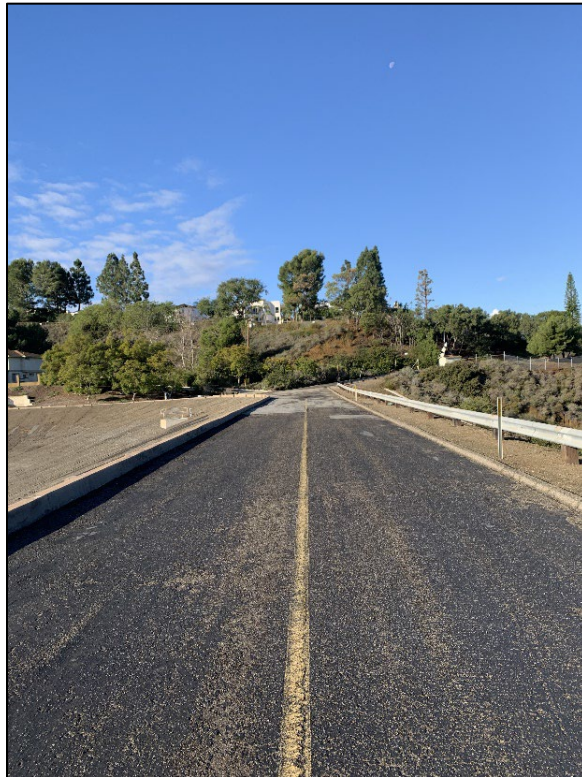
Photo 3) AC paved crest looking towards the left abutment.
