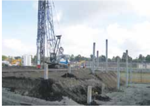
Out with the old and in with the new: The above photo chronicles the demolition of Michelson Water Recycling Plant's phased-out aeration basins. The photo below depicts the same site with pile driving in production for the new membrane bio-reactor.
