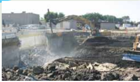
Out with the old and in with the new: The above photo chronicles the demolition of Michelson Water Recycling Plant's phased-out aeration basins. The photo below depicts the same site with pile driving in production for the new membrane bio-reactor.
