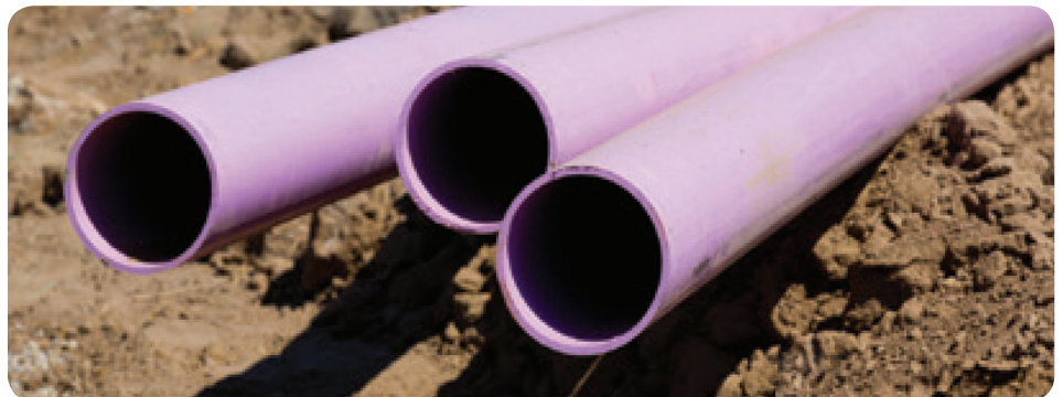
IRWD uses purple pipe throughout its recycled water system to identify the presence of recycled water. This helps ensure recycled water is always kept separate from drinking water.
