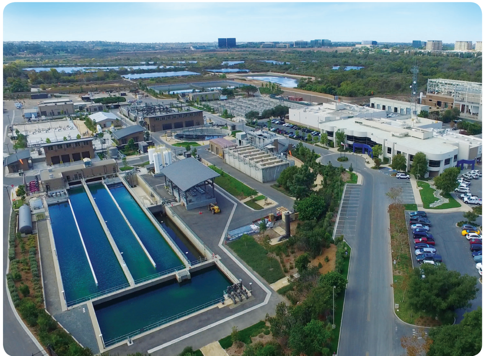
Michelson Water Recycling Plant aerial view shows chlorine contact disinfection tanks in foreground.
