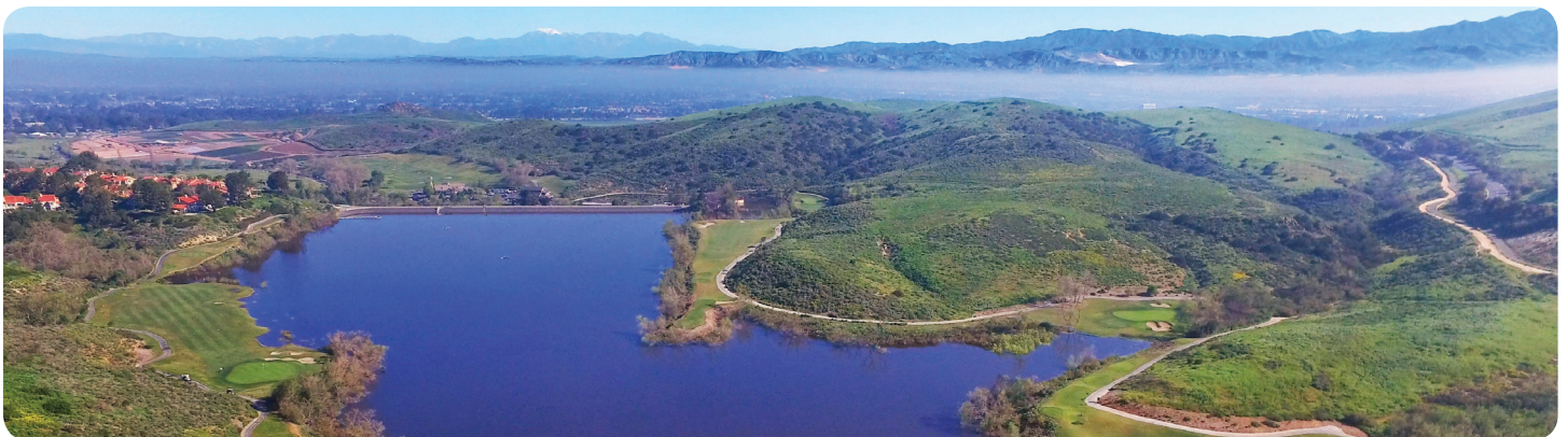
Storage capacity is vital to a recycled-water system. Sand Canyon Reservoir—adjacent to the Strawberry Hills golf course in Irvine—has a surface area of 42 acres, an average depth of 18 feet and a volume of 250 million gallons. The picturesque reservoir is used for both seasonal and operational storage.
