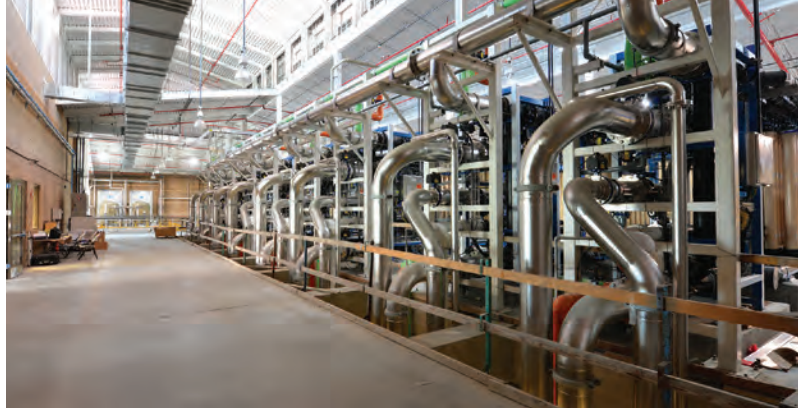
Baker Water Treatment Plant
