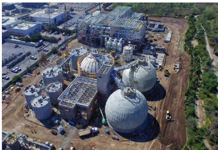
Biosolids and Energy Recovery Facilities Project
