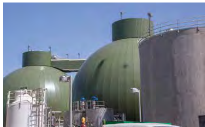
Biosolids and Energy Recovery Facilities Project
