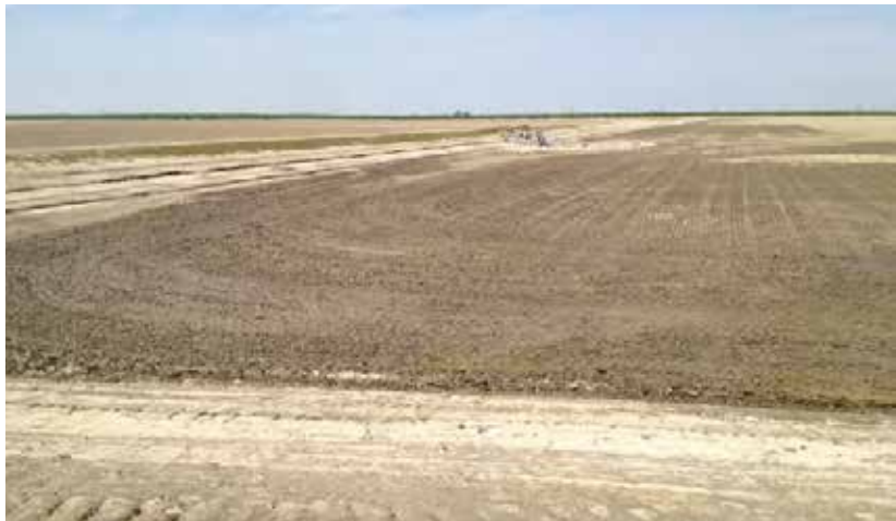
View of existing Stockdale West recharge basin
